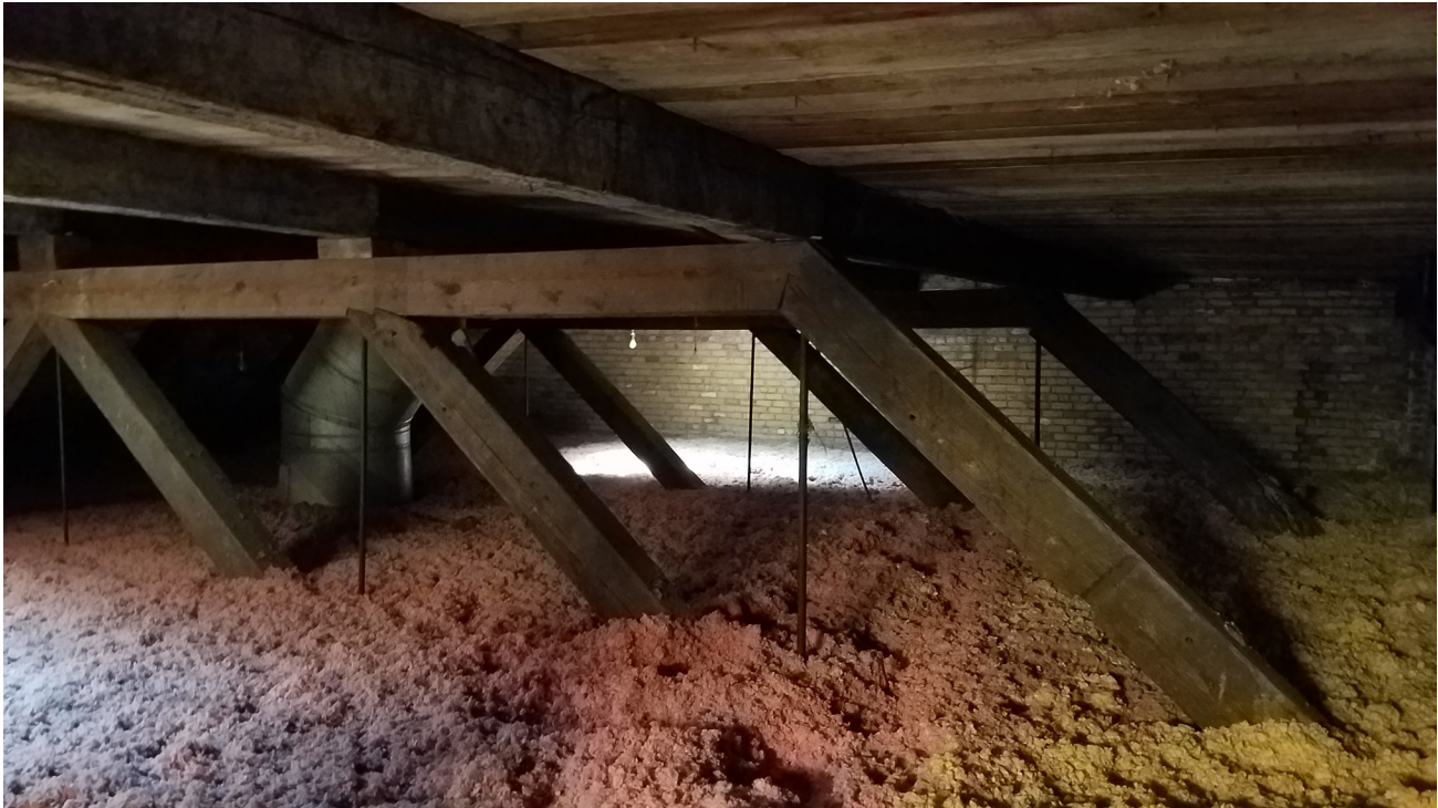
Attic, showing wood trusses and loose fill insulation.
