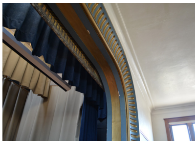
Jamb of the proscenium arch.
