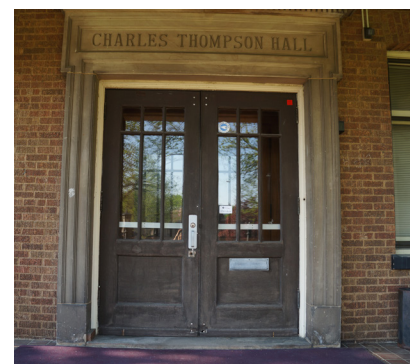
North entrance doors beneath porch.
