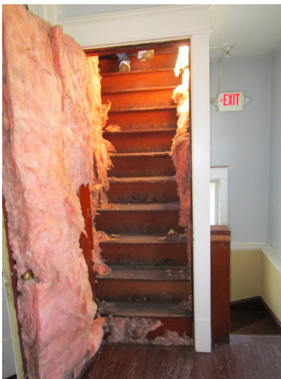
Stairway to the attic from the third floor hallway.
