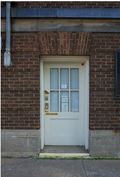
South entrance door.
