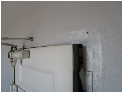
Top of projection room door and frame behind the plaster.
