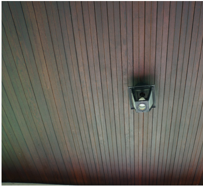
Dry porch ceiling.
