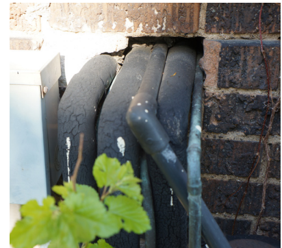
Pipe penetrations in brick at east facade.
