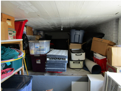
Storage room underneath the stage.
