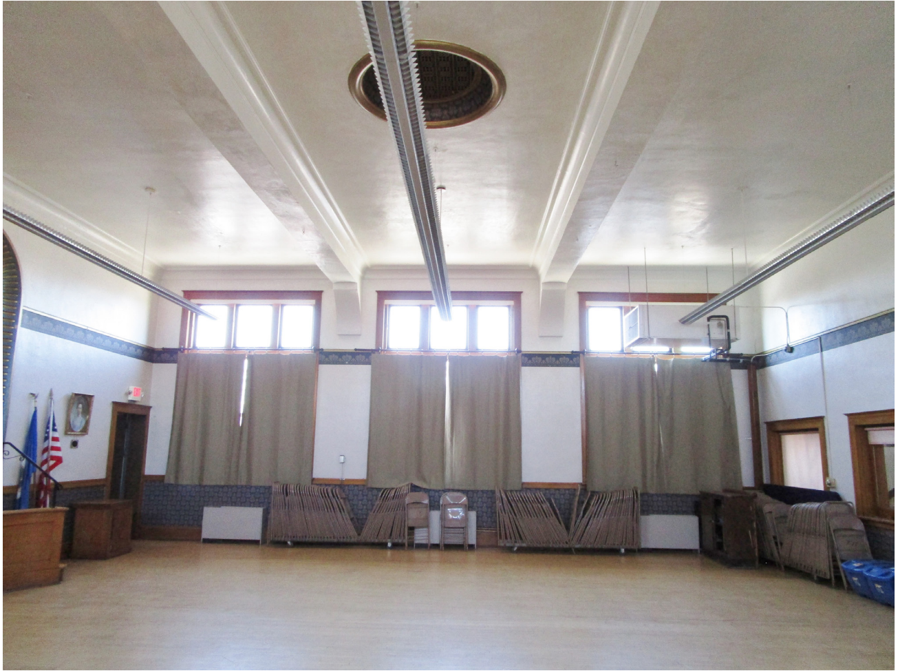
View of the Assembly Hall's large ceiling beams and windows, facing east.
