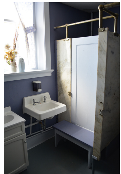
Sinks and bench in front of stall in the women's toilet room.
