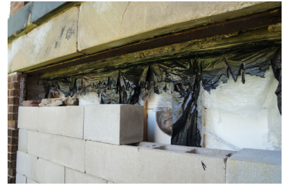
Partially completed infill of opening below porch.
