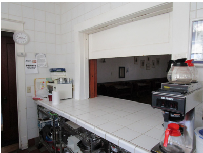
Kitchen counter and passthrough to the dining room.
