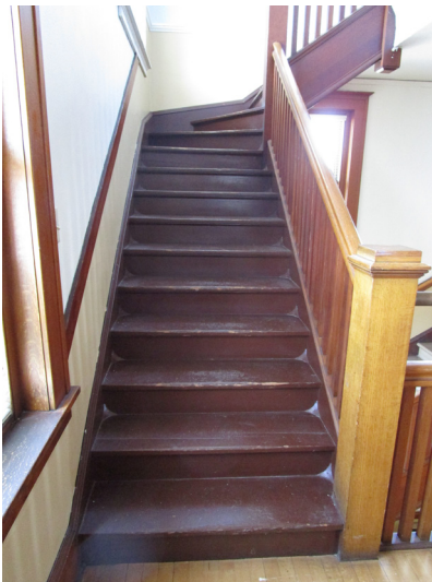
Stairs from the second floor to the third floor.
