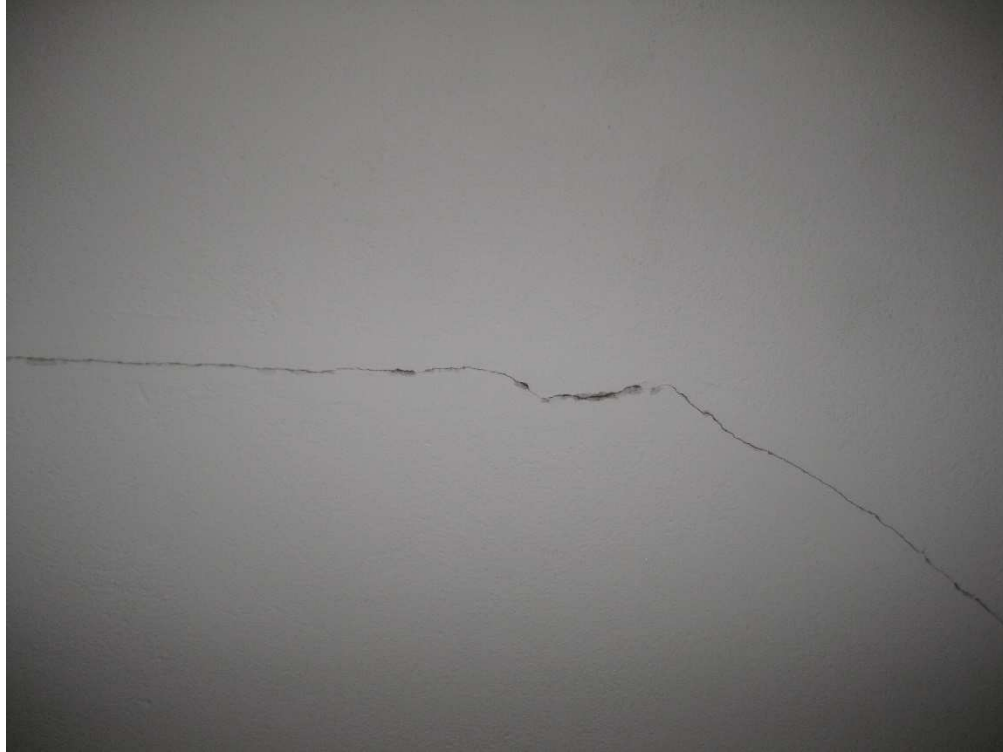
Photo 5 - Third Floor Printing Room ceiling
