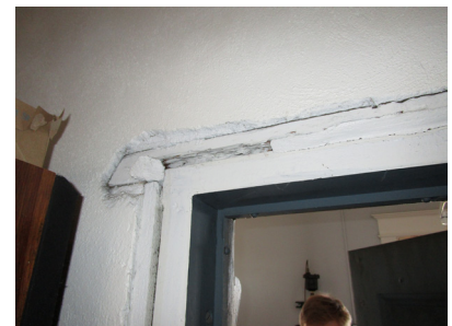
Top of door frame in the Moving Picture Operating Room.
