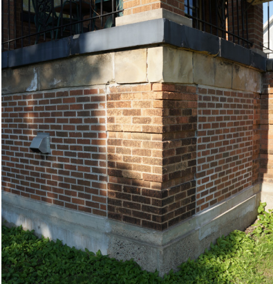
East porch openings that have been infilled with brick.
