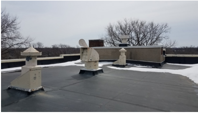
Photograph of the roof, facing southeast.
