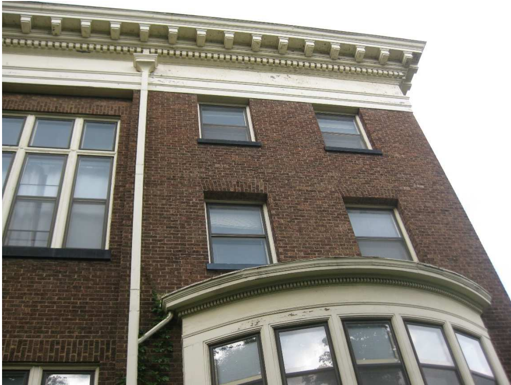
Photo 9 - East Elevation - near bow window
