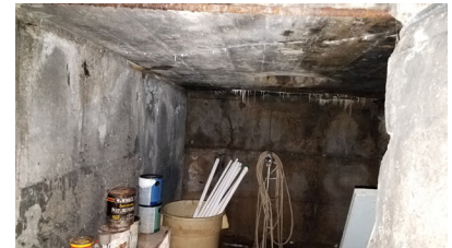
View into the ash bin and coal room.
