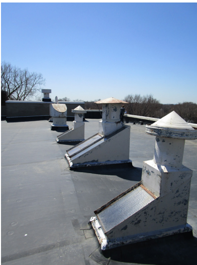
Skylights and vents along the center of the roof.
