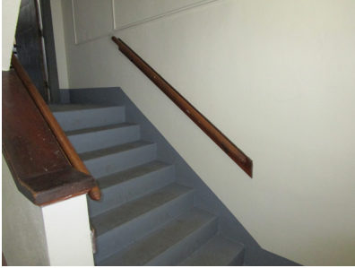
Photograph showing handrails.
