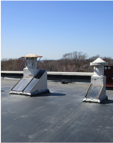
Skylights at north side of roof.
