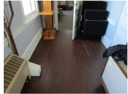
Third floor hallway.
