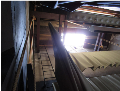
Fly loft and view of ladder on the south stage wall.
