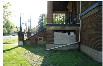
East side of the porch.
