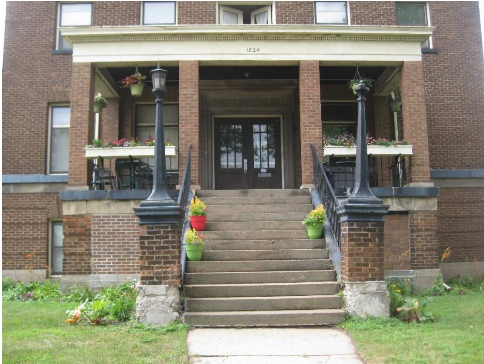
Photo 13 - Front stairs / porch
