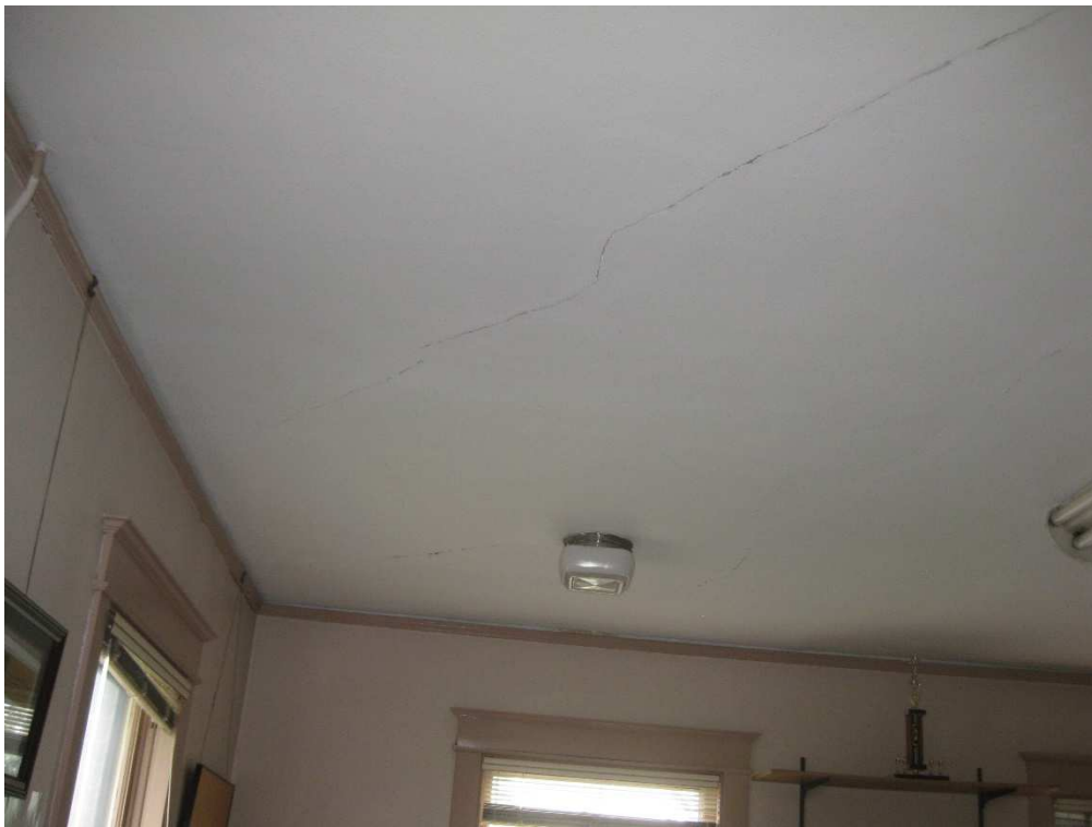
Photo 4 - Third Floor - Printing room ceiling
