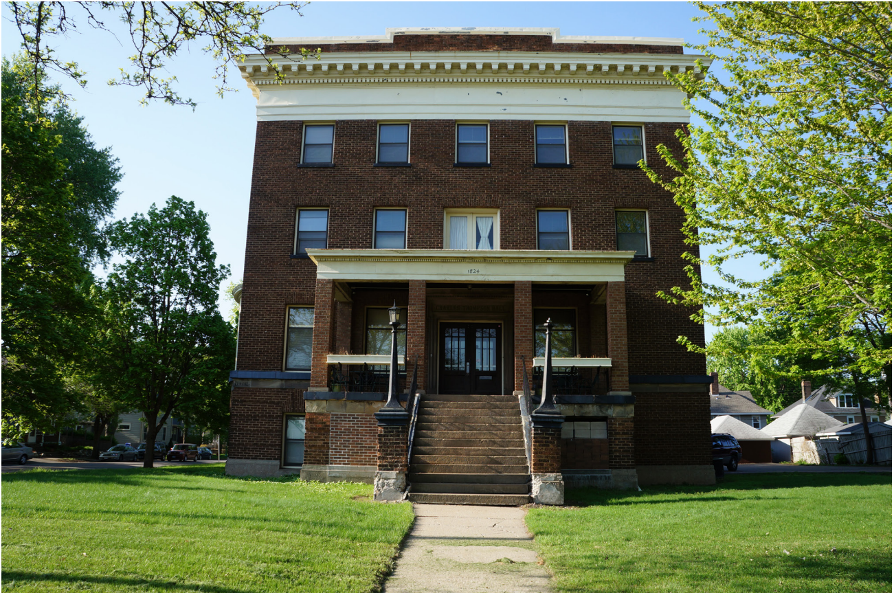
North facade of Charles Thompson Memorial Hall.
