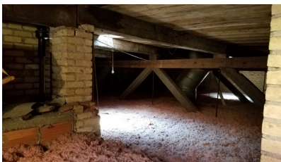
Photograph of the attic space.
