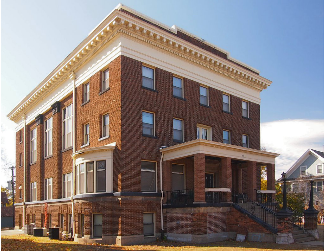
View of the northeast corner of Charles Thompson Memorial Hall.
