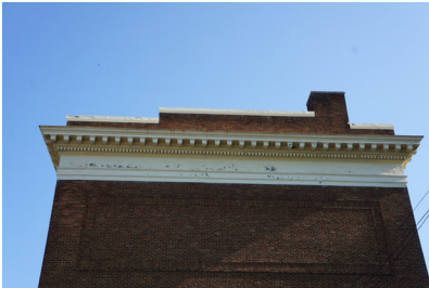
Rectangular brick pattern at the top of the south facade.
