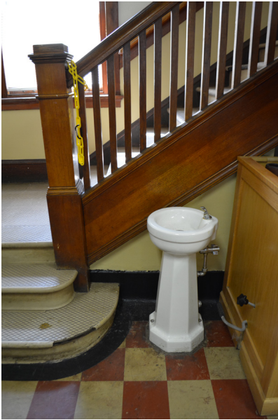
Drinking fountain by the front stairs in the basement.
