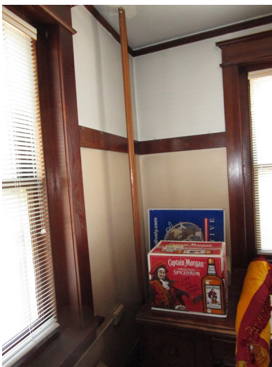
Pipe penetration in corner of Coat Room.
