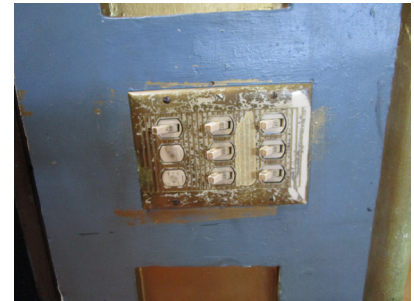
Light switches in jamb of proscenium arch.
