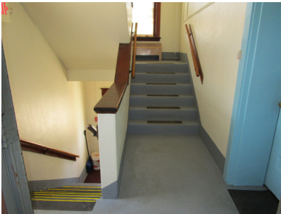
First floor landing of the back stairs, adjacent to the apartment.
