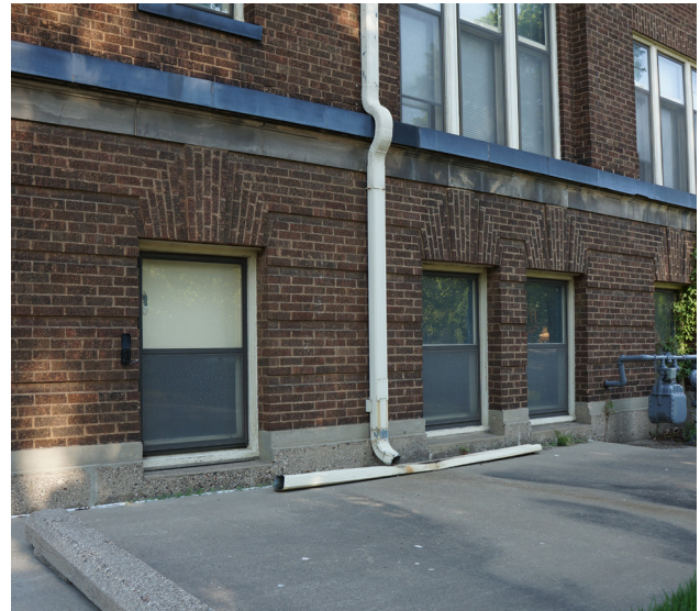
South downspout on the east facade.
