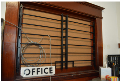
"Office" sign and boarded up window with metal bars in Committee Room.
