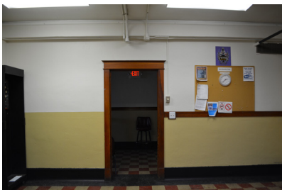
Missing trim to the left of the door to the main hallway in the Card Room.
